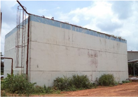
Figure 7. Plant in S2, bio-digester
