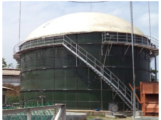
Figure 6. Plant in S1, bio-digester
