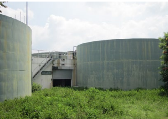
Figure 9. Plant in P2, bio-digester
