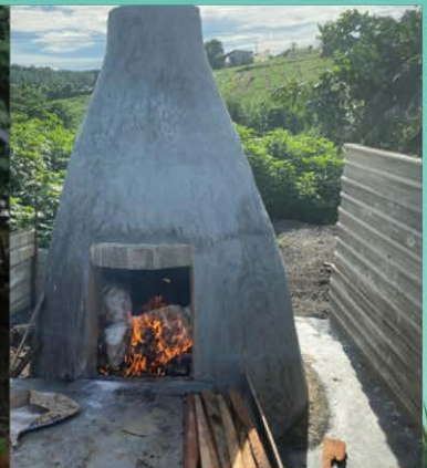
Gambar 6: Incinerator bata sumber: (Ladang Lida, Johor)
